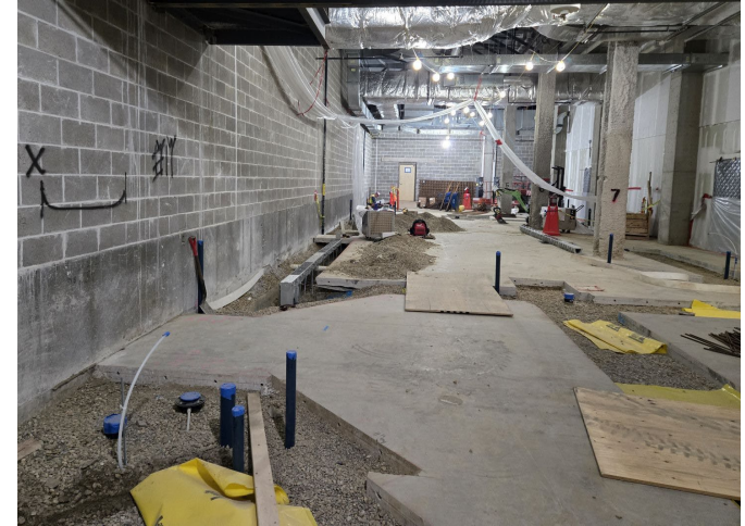
Slab demolition and utility installation
