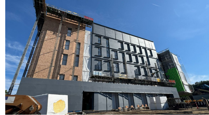
Exterior Sheathing and Finishes
