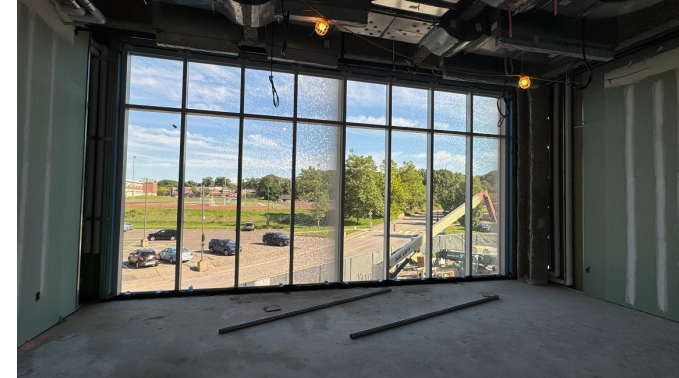
Interior Walls and Window Assembly
