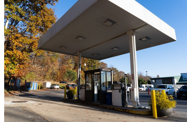
Existing Conditions at Dispensing Facility
