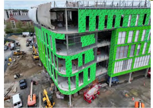
Exterior Framing and Sheathing
