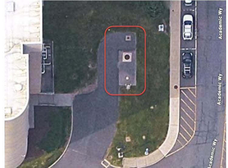
Aerial view of existing tank location
