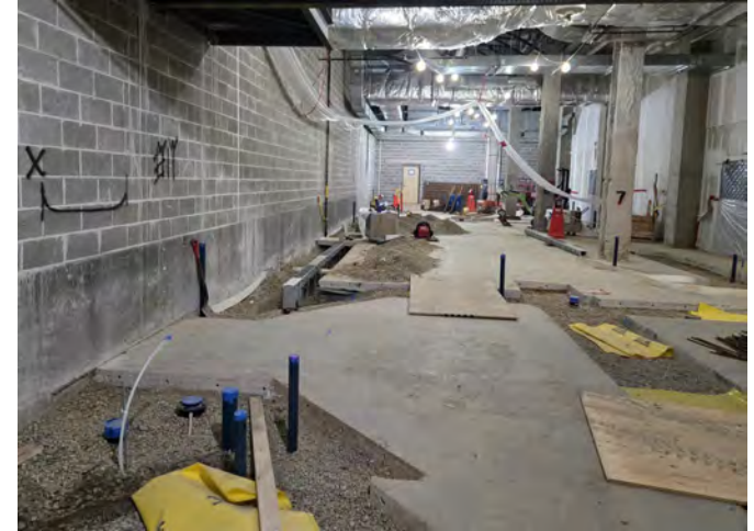
Slab demolition and utility installation
