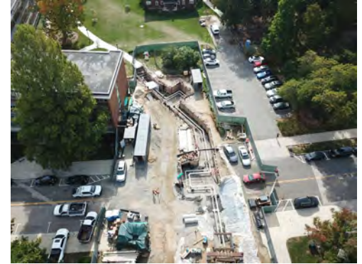
Steam Installation Prior to Site Restoration
