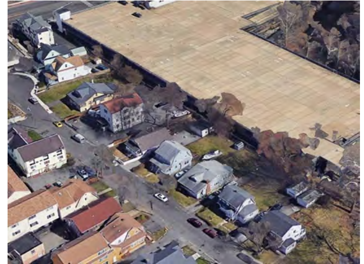
Vernon Place neighborhood prior to demolition of garage
