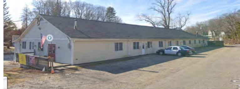
Existing ~10,000 SF building to be demolished
