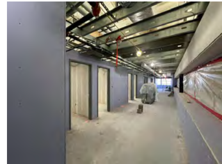
Second floor Offices
