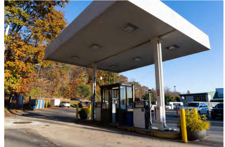
Existing Conditions at Dispensing Facility
