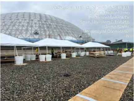
Roof Panel Prep Area
