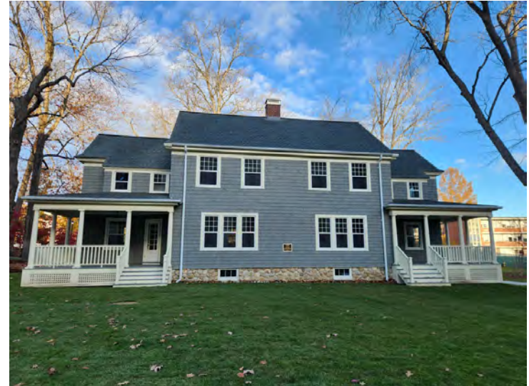
4 Gilbert Road - House Relocation
