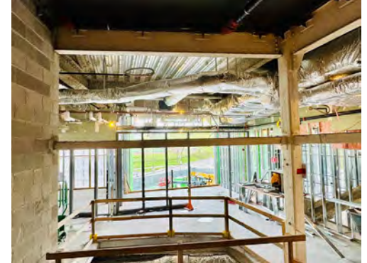
Interior Framing and Mechanicals
