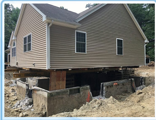
$200K+ Foundation Replacement
