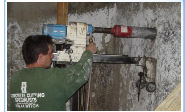
Concrete Cores from Homes
