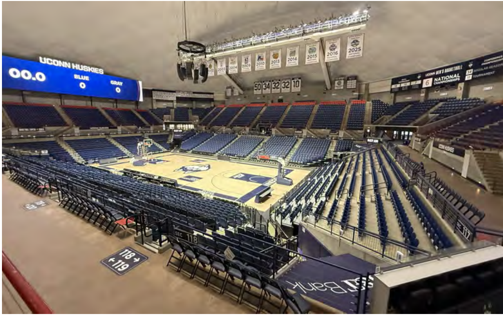
Bleacher Seat Installation
