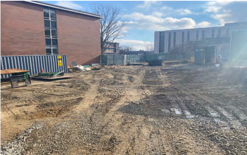
Steam line work completed and backfilled
