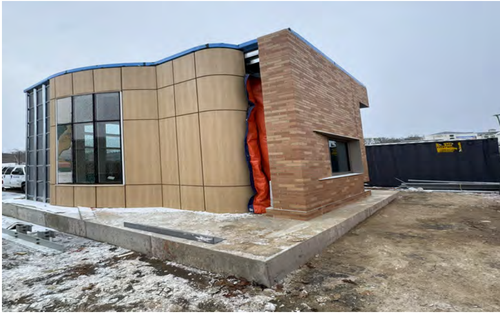
Mockup (partial construction of Exterior Elevation)
