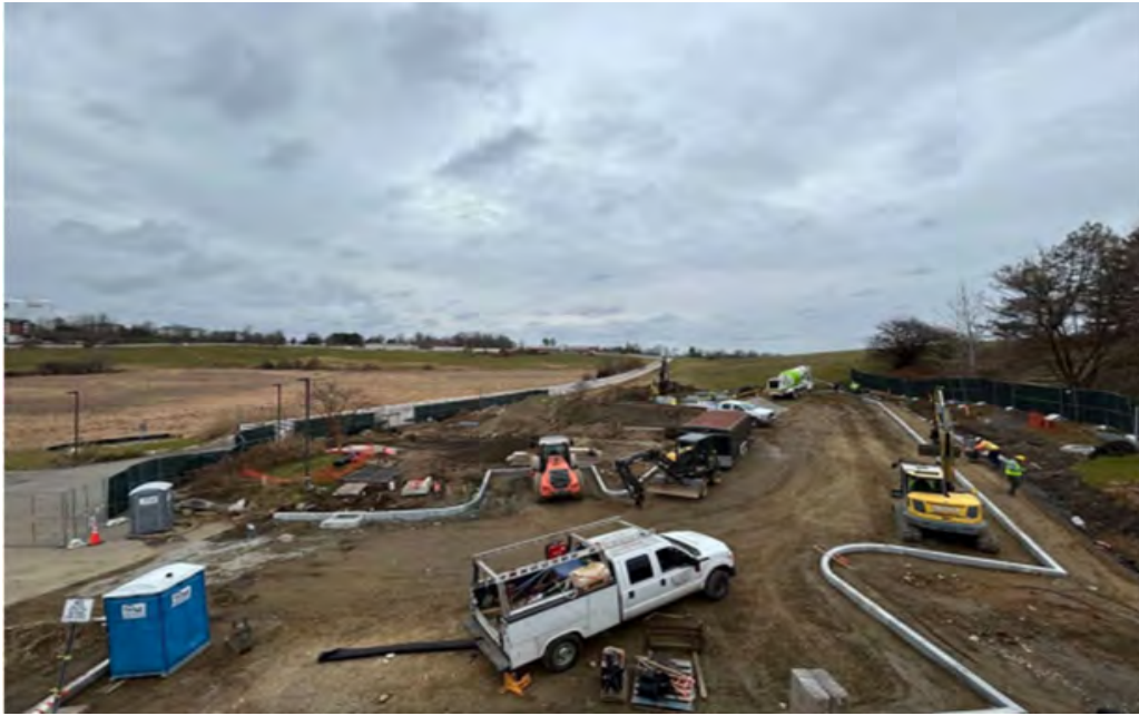
Jones Annex – November 2025 Upper Parking Lot
