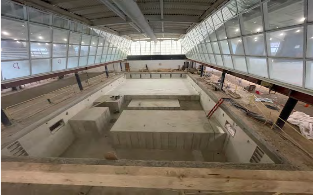
Phase II - Hydrotherapy Tanks Footing Blocks in Place
