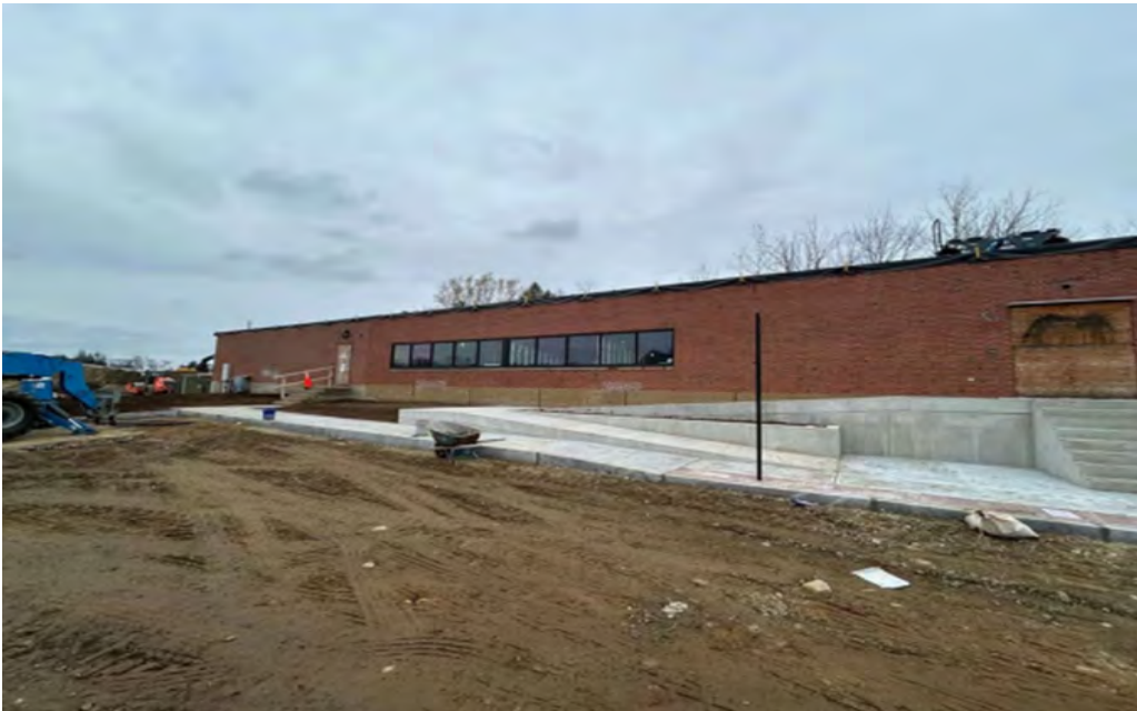
Jones Annex – November 2025 Front of Building
