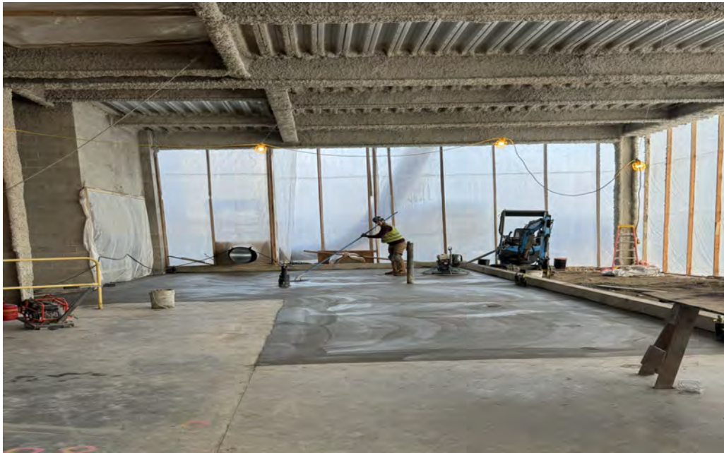
Interior concrete slab and fireproofing on steel above
