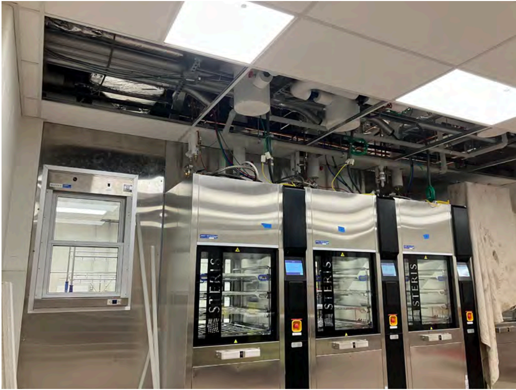
Steris Washers – Installation of New RO Water and Domestic Water Piping
