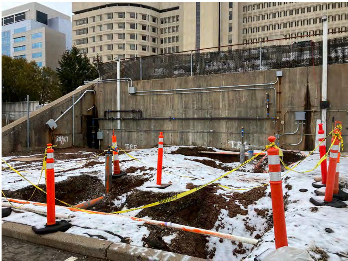
Old Oxygen Pad Removed and Test Pits Dug
