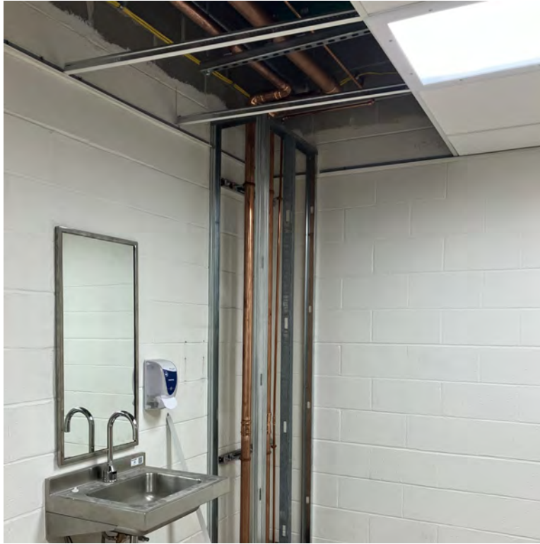
Installation of New Domestic Water Supply in CB011F from H-Subbasement
