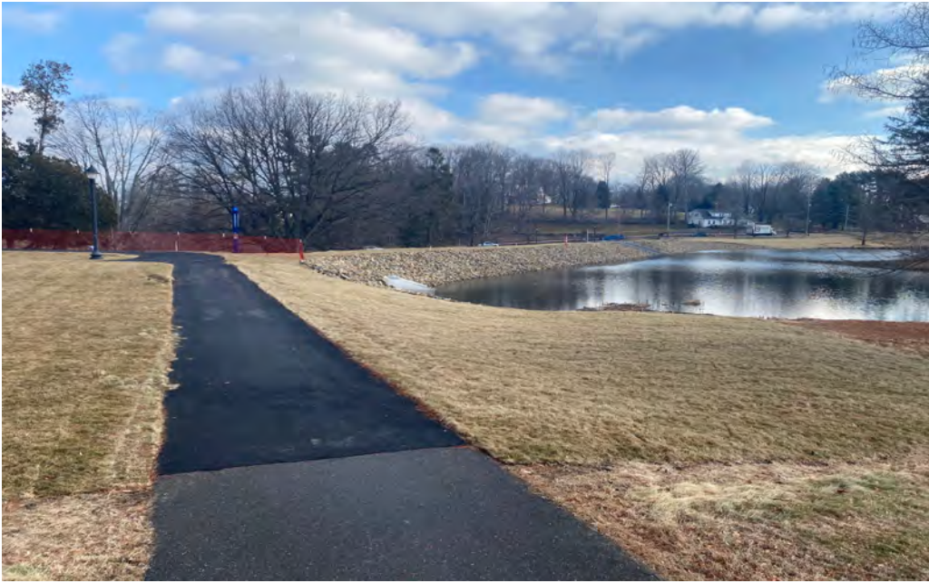
Completed embankment and spillway
