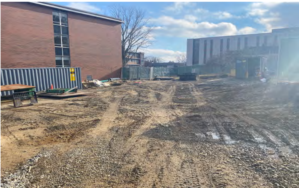
Steam line work completed and backfilled
