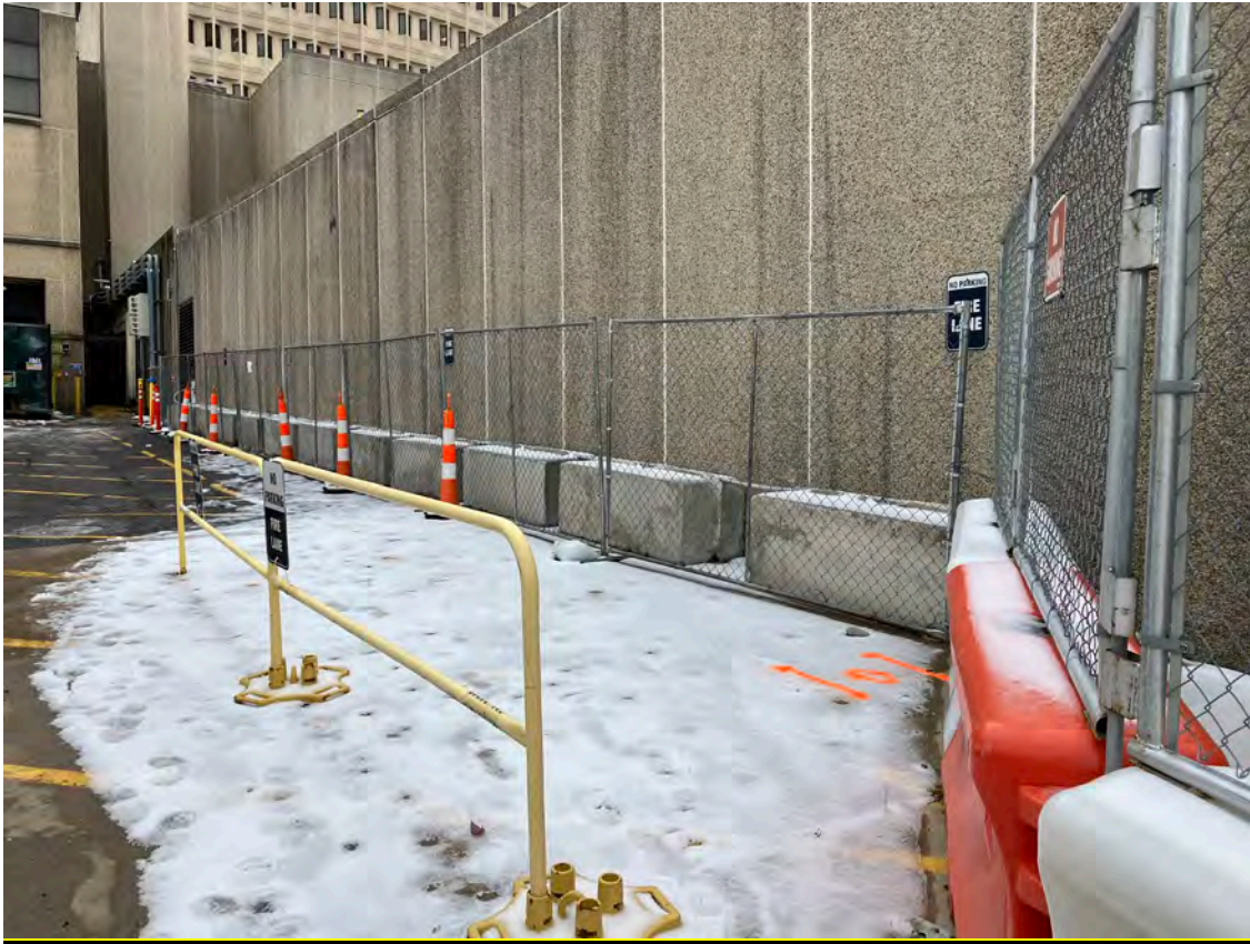
Second Temporary Oxygen Line Run to Main Building
