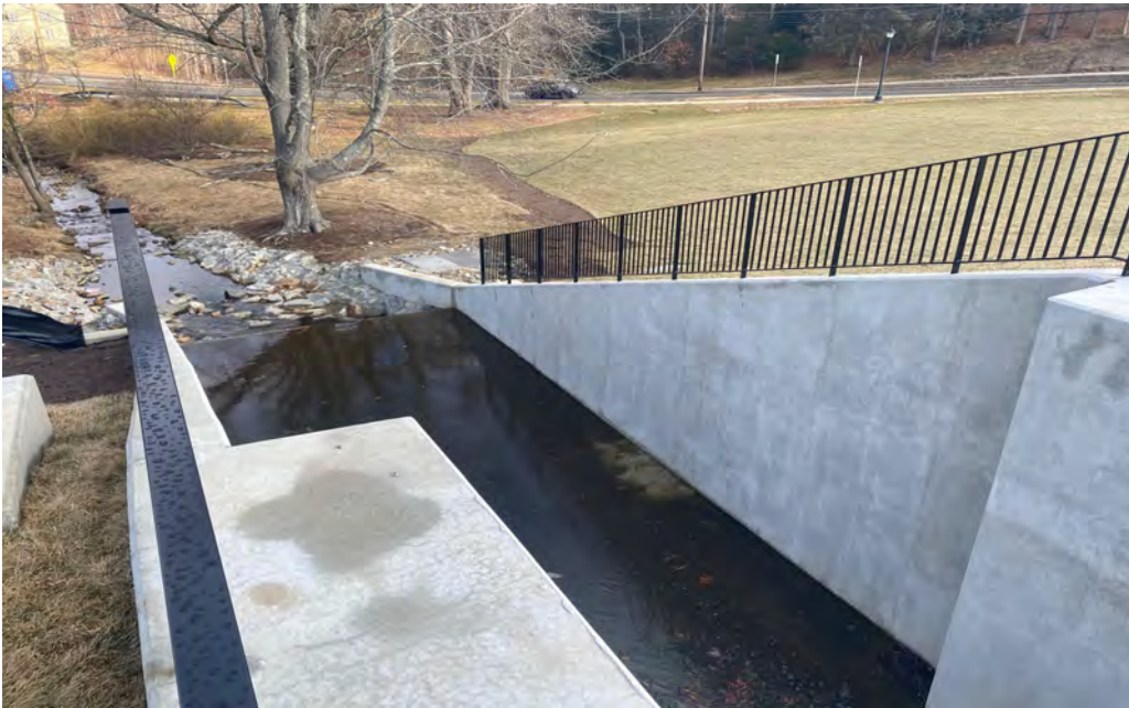
Completed spillway looking downstream
