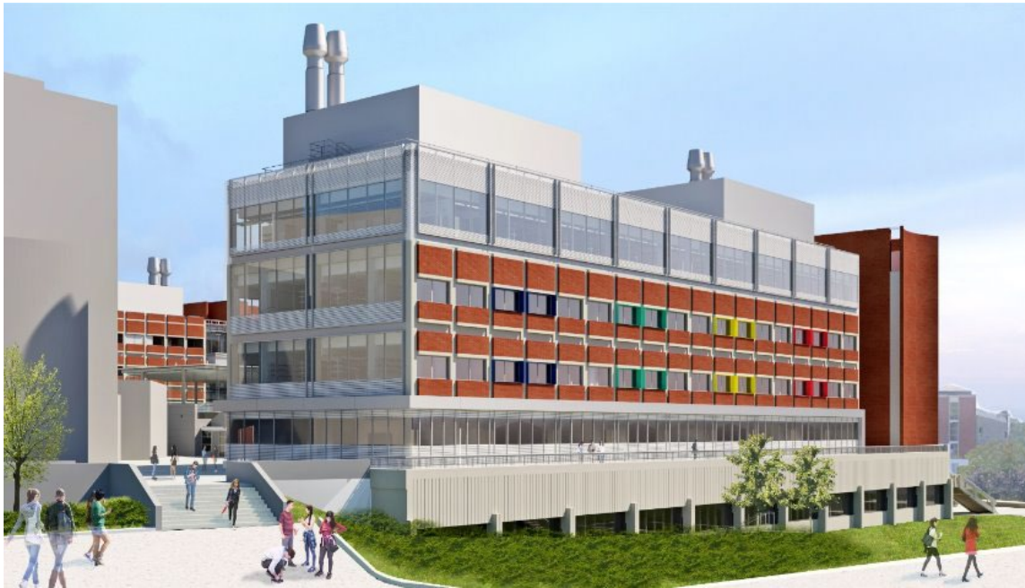
View of 4th Floor North Wing Addition from North Eagleville Road
