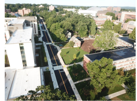
Completed utility installation and restored Gilbert Road
