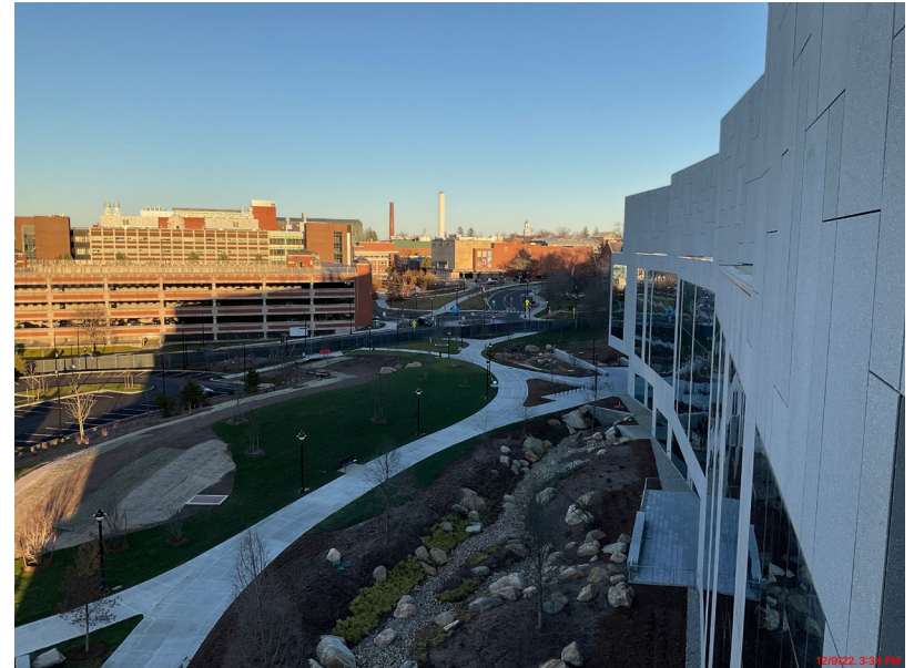
North Elevation Looking East
