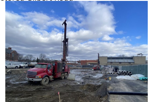
Installation of geothermal system, S Lot
