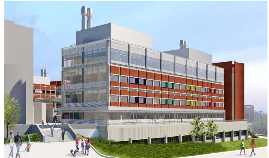
View of 4 th Floor North Wing Addition from North Eagleville Rd
