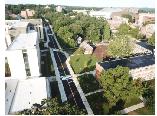
Completed utility installation and restored Gilbert Road
