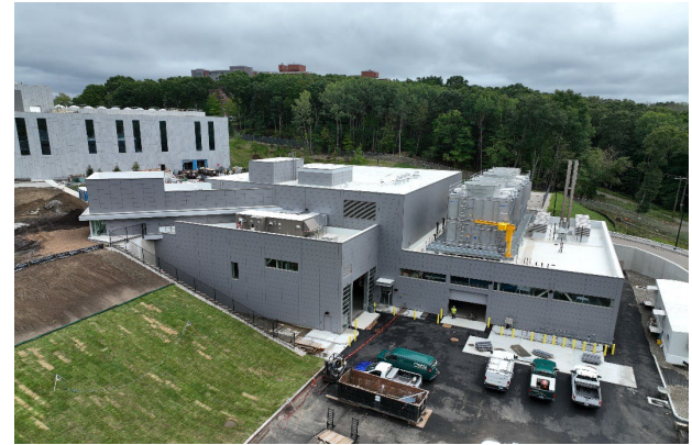
SUP View Looking South
