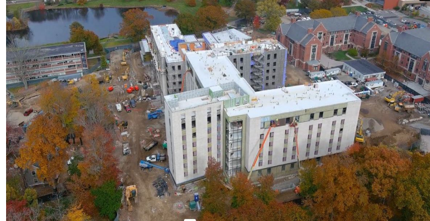
View looking southwest of construction on the two L-shaped wings of the Residence Hall
