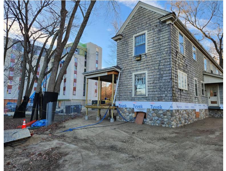
4 Gilbert Road - House Relocation
