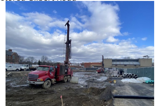
Installation of geothermal system, S Lot 10
