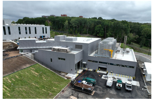
SUP View Looking South
