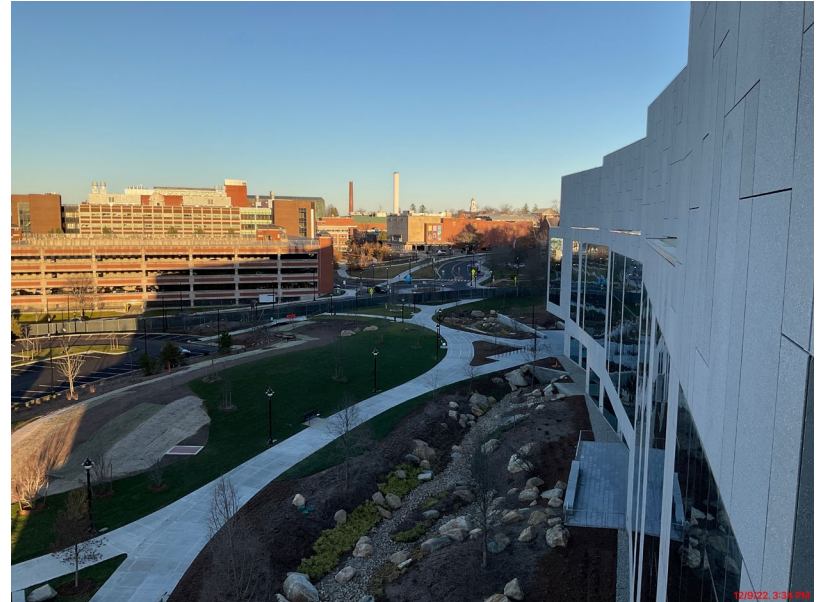
North Elevation Looking East
