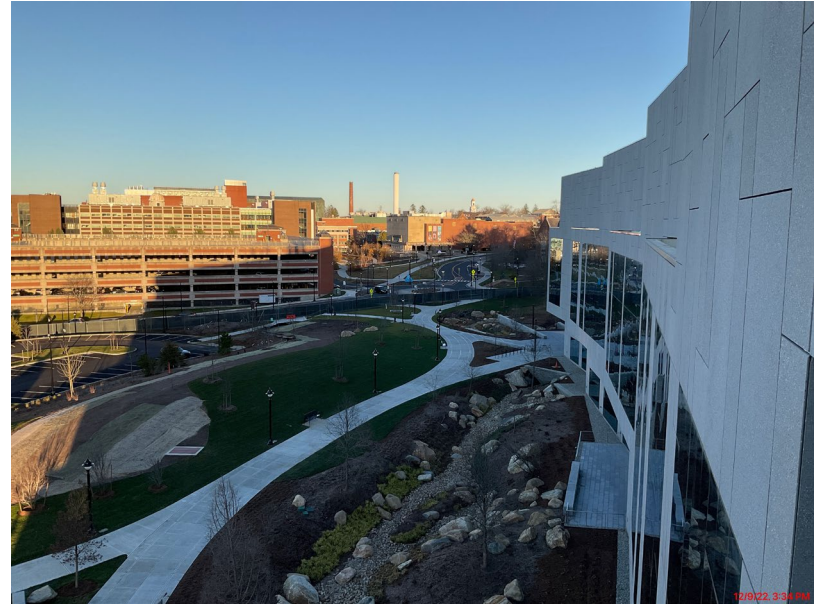
North Elevation Looking East
