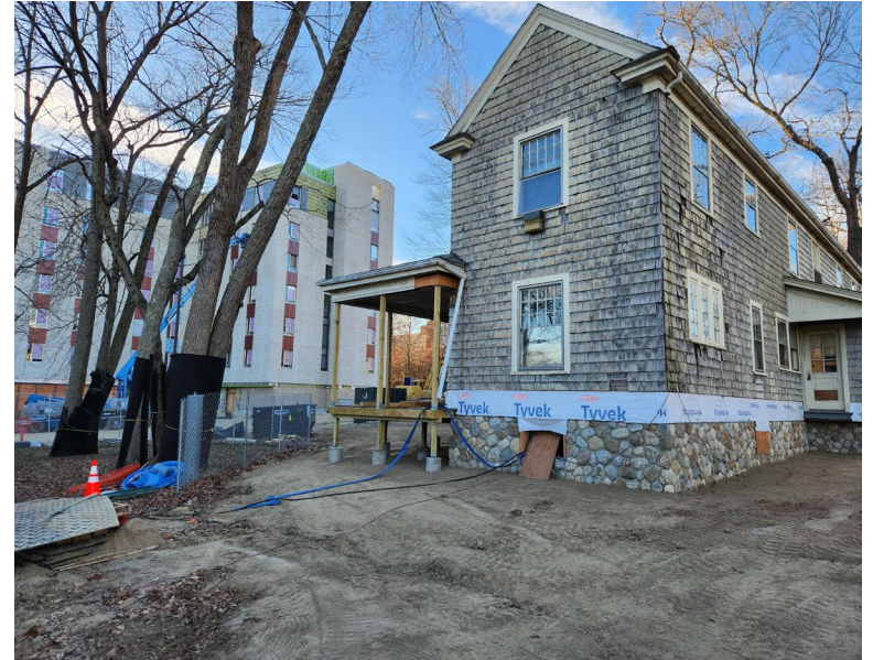
4 Gilbert Road - House Relocation
