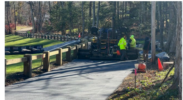
New Roadway being installed
