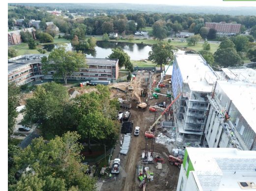
Installation of new utilities in Gilbert Road
