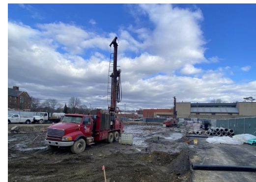
Installation of geothermal system, S Lot 10
