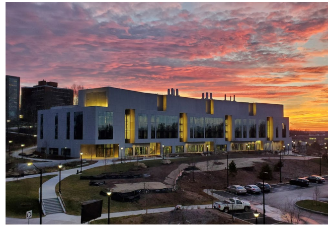
North Elevation Looking South
