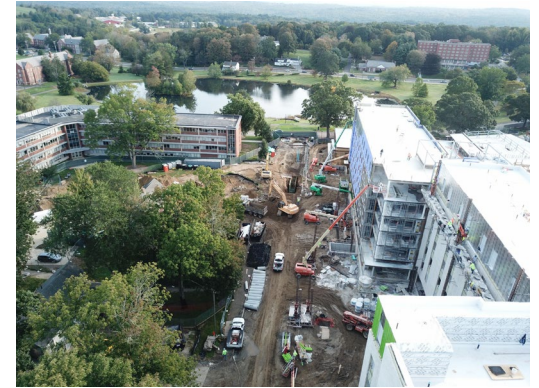
Installation of new utilities in Gilbert Road
