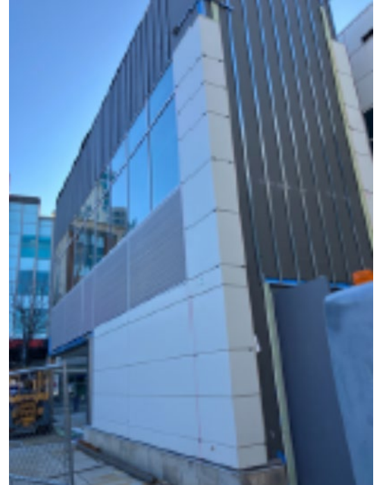
New Exterior Stairwell at West Side of Building
