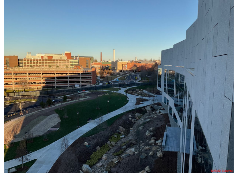
North Elevation Looking East
