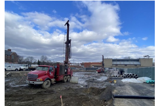
Installation of geothermal system, S Lot
