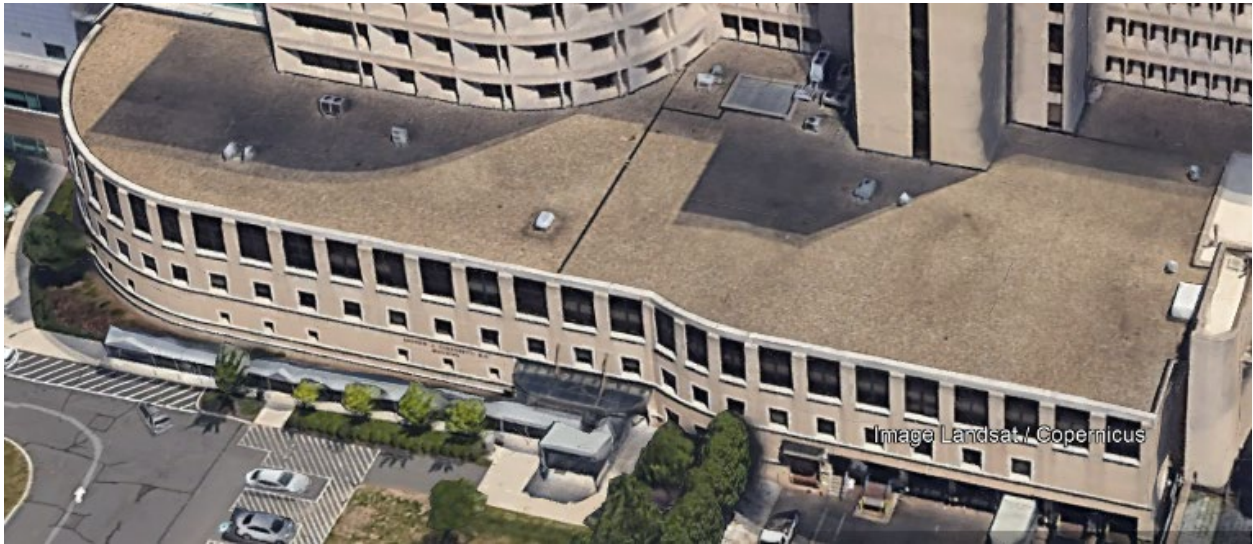
BUILDING F (CANZONETTI BUILDING) ROOF
