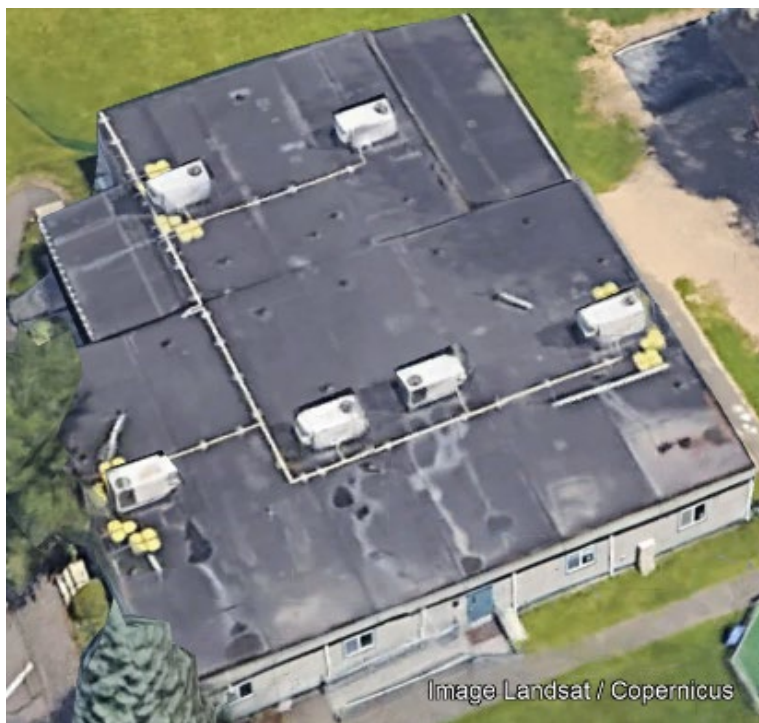
BUILDING M (DAYCARE CENTER) ROOF
